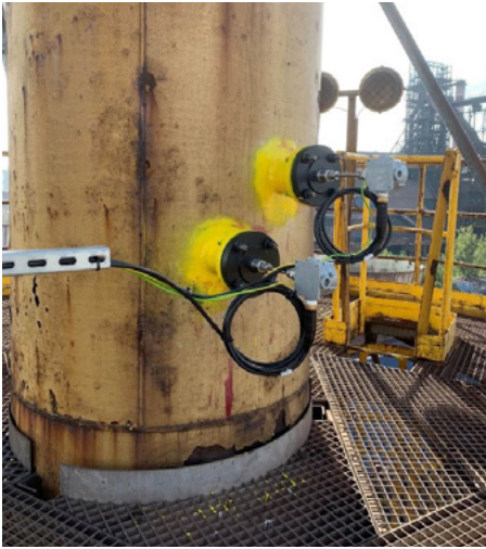
Picture 11. Combustion chimney with a T5 bias 90 setup on a DN1200 (48") pipe for blast furnace gas
