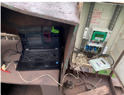
Picture 1. Replacement of AT868 flow meters on the Coke oven battery.
